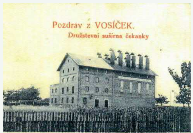
Figure 3. A dryer company building in Osíčky on a historical postcard.
